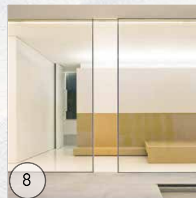
8 LOW IRON GLASS WITH BLACK ALUMINUM FRAME
