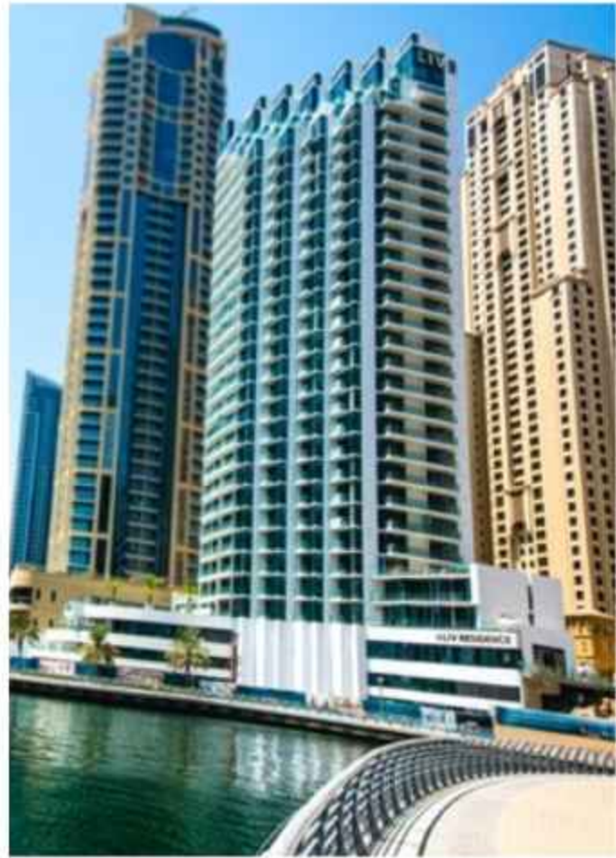
LIV Residence COMPLETED & HANDED OVER
