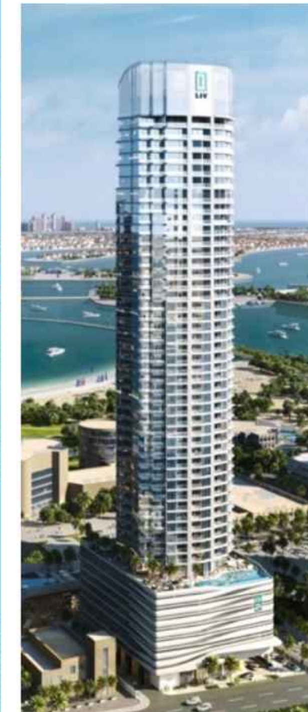
LIV LUX CONSTRUCTION IN PROGRESS HANDOVER 2026
